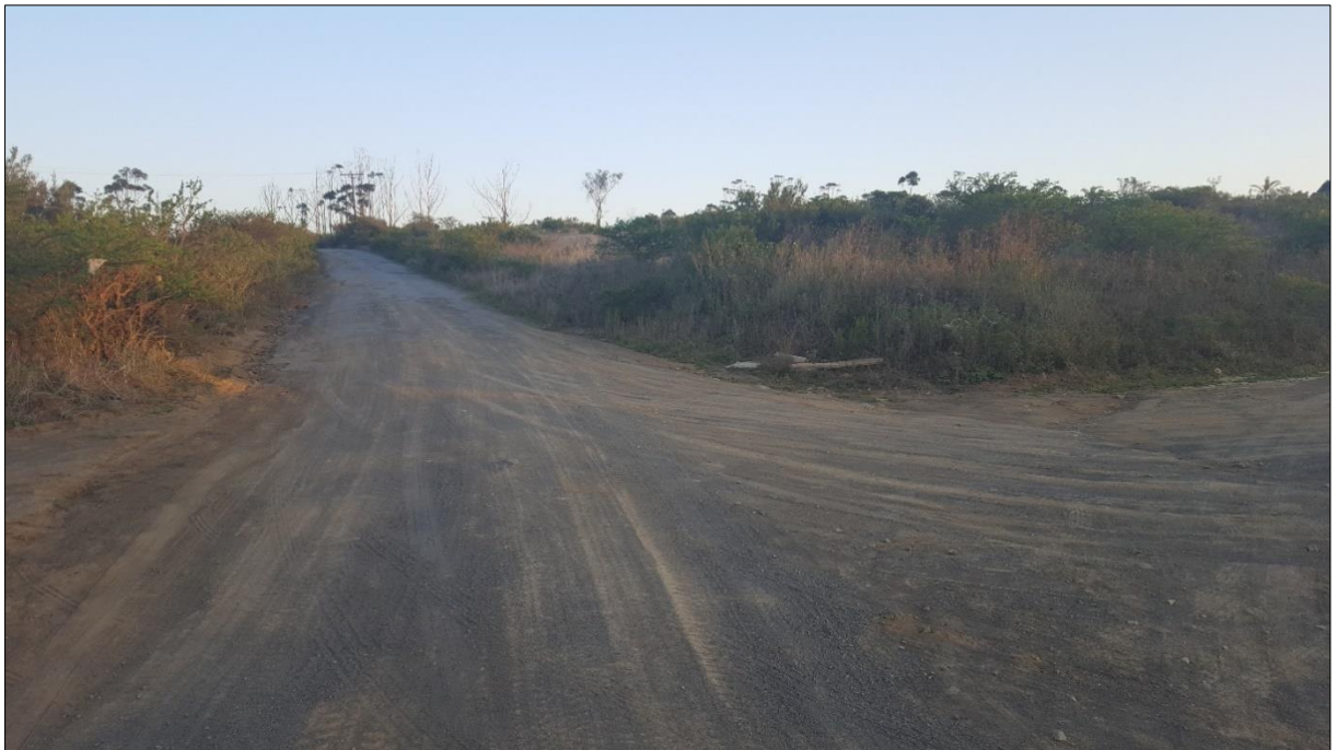
Photo 4-3: Road B leg, in direction of R102
